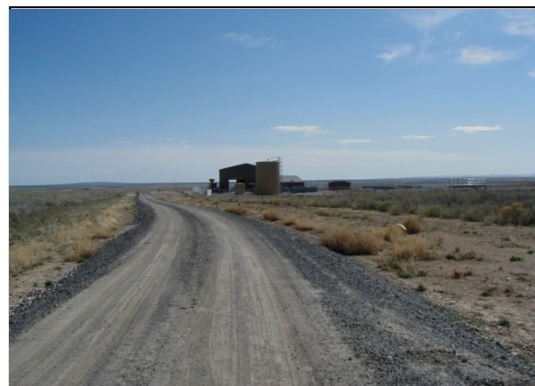
Juniper Butte Range Operations and Maintenance Complex
