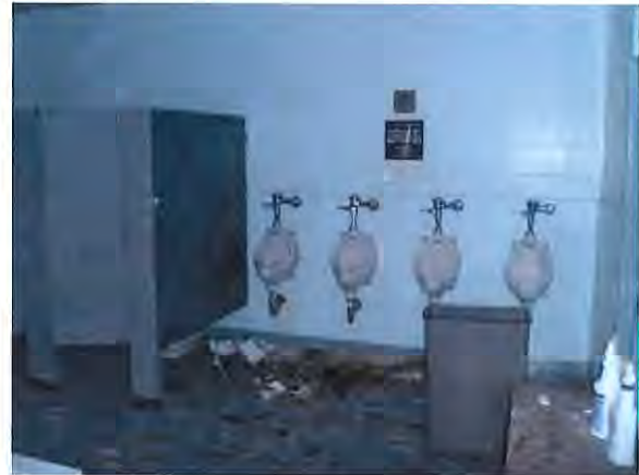
Figure 2-8: Rodent infestation at Men’s restroom
