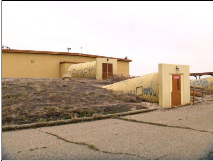
Photo 3.7-2. View of the Exterior of the Ramped Entrances.
