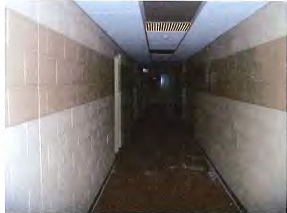
Figure 2-4: Typical interior lower level corridor
