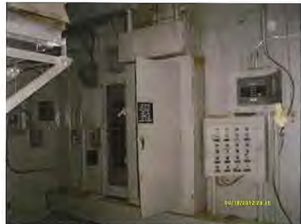
Figure 2-9: Main electrical panel at mechanical room
