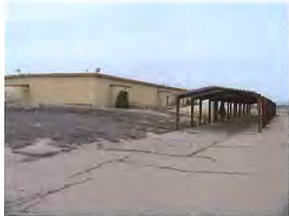
Figure 1-1: Exterior view from the southwest
