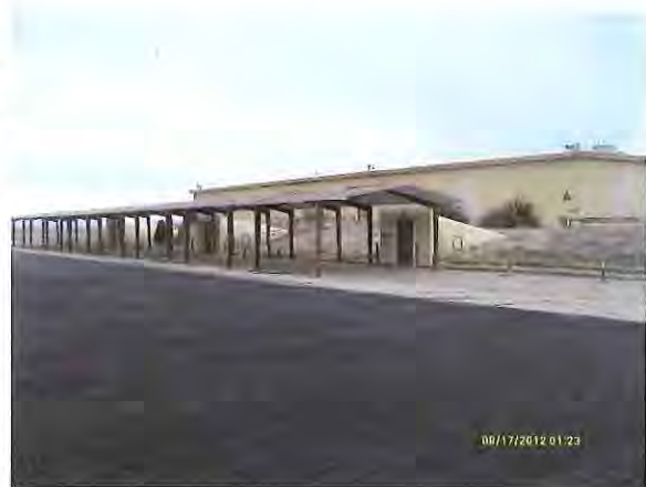
Figure 2-6: Exterior view from the southeast
