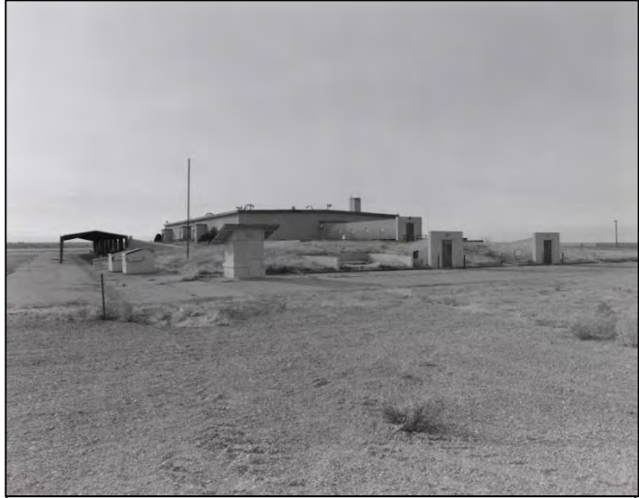
Photo 3.7-1. General Overview of Building 291, Facing North (Taken from MHAFB 2013).
