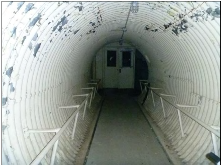
Photo 3.7-3. View of the Interior of the Ramped Entrances.
