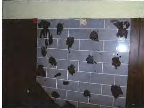
Figure 2-1: Asbestos mastic used for wall paneling
