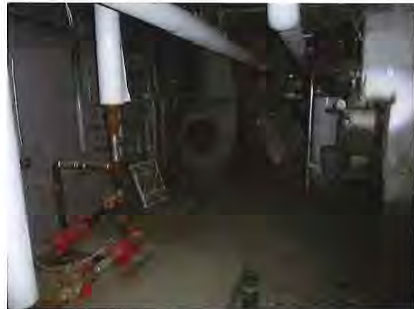
Figure 2-7: Mechanical room at lower level
